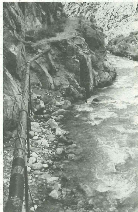
Damage to the North Kaibab Trail and water pipeline caused by flooding in March 1995. Grand Canyon National Park photograph.
